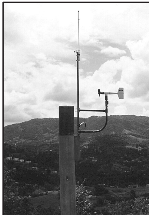
Weather Sensors retrofitted to an existing rain station in Puerto Rico.
